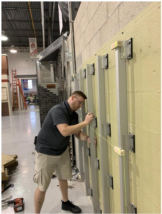
6. Now secure the rest of the mullions to the girts using the remaining 1 <sup>1</sup>/<sub>8</sub>" screws as you did in step #4.
