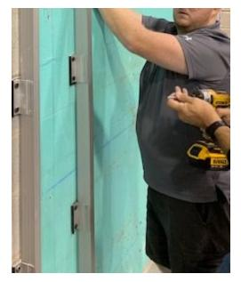
2.2. At this point set only one fastener at the top of each girt along a given wall spacing, such as a twelve foot span. Once all of the mullions are 'hanging', use a six foot level to plumb the girt/mullion assembly and then set it in place by putting a fastener in the bottom of each girt.
