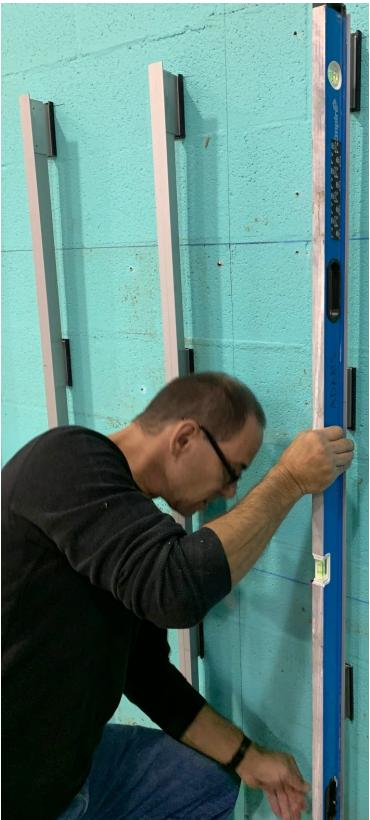
5. Once your two outside mullions are in proper position, use 3' string blocks' and some string to align the top, middle and bottom of all the mullions in between the left and right from the previous step. As before, just pull or push the mullions into position using the string as a guide to align the face of the mullions.
